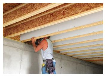
Installing 1/2-inch gypsum board to I-joist webs is one of several methods builders and installers can use to meet the IRC provisions.
