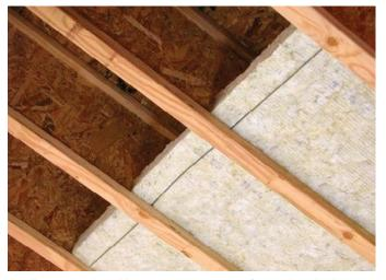
Installing mineral wool between I-joists is one of several methods builders and installers can use to meet the IRC provisions.
