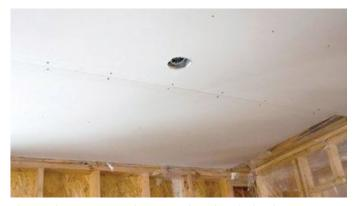
The IRC does not require the gypsum board applied to the underside of the I-joist floor systems to be covered with tape and joint compound.
